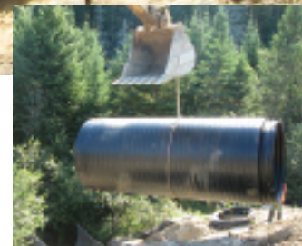
78"ID Weholite pipe is lowered into place.
